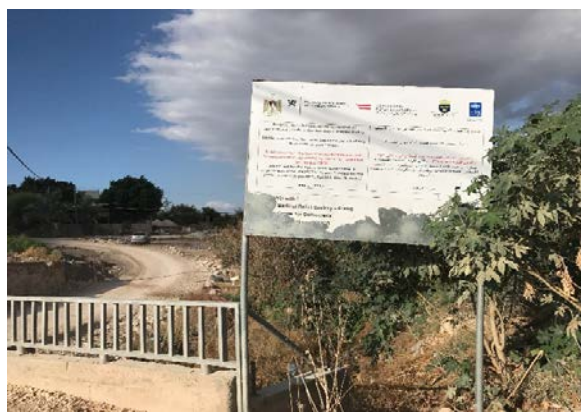
Figure 11: A section of agricultural road that was rehabilitated in Tubas cluster
